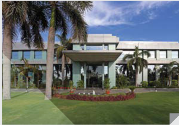
Harsha Engineers International Limited, Changodar Plant, India
