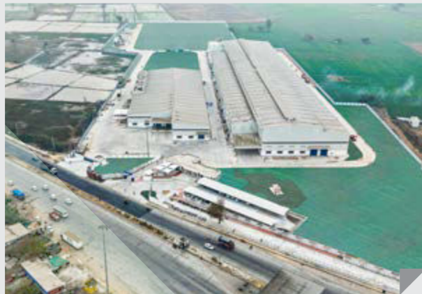
Harsha Engineers Advantek Limited, Bhayla Plant, India
