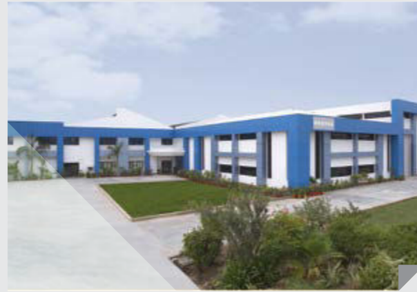
Harsha Engineers International Limited, Moraiya Plant, India
